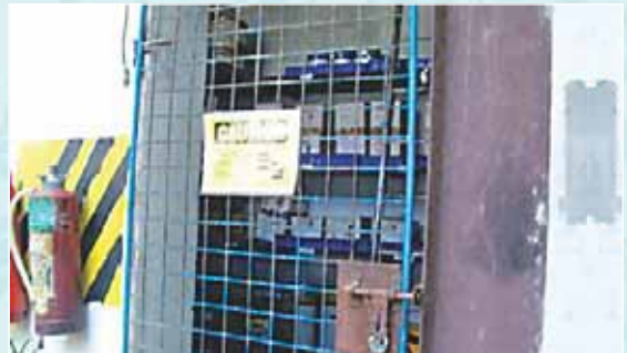
Chemical Storage Area- Caution Signage, Fire Extinguisher Nearby
